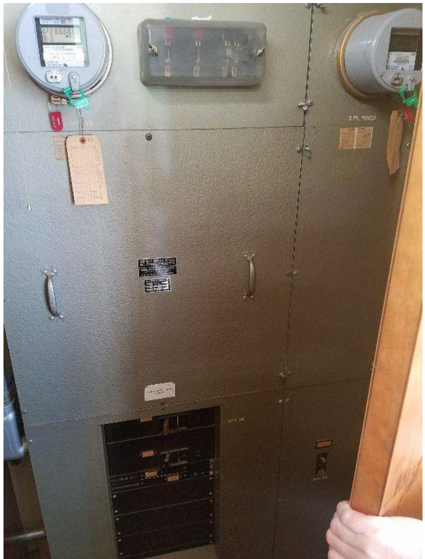
This is in the upstairs office closet area.
